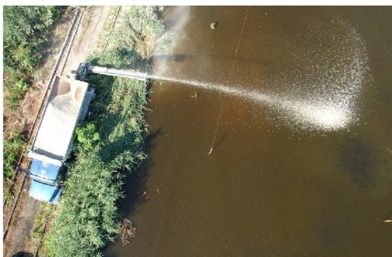
One approach to cap construction, i.e. a land-based, truck-mounted conveyor (source: AquaBlok, Ltd.).
